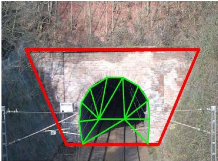
Figure 7: TIC (the opening's outer ring (green) and the triangulated ClosingSurface (green TINs).
